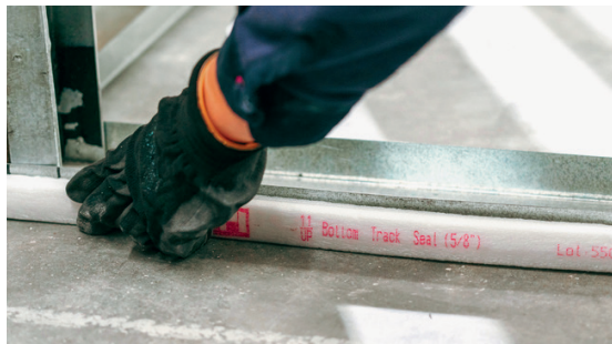
Fig. 27: Bottom track seal installed on floor runner
