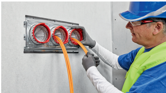
Fig. 10: Speed sleeve with gang plate, Hilti CFS-SL GA used for small cable bundles
