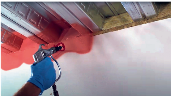
Fig. 28: Hilti CFS-TTS MD installed correctly per EJ
