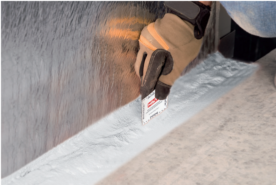
Fig. 33: Correct depth of sealant, Hilti CFS-SP SIL
