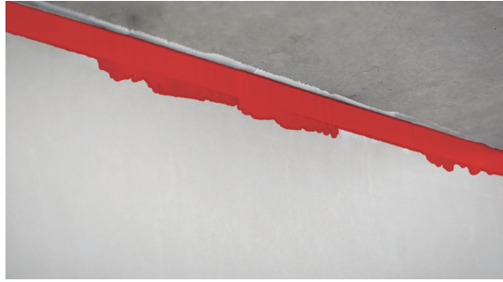
Fig. 23: Firestop sealant applied to the top-of-wall joint
