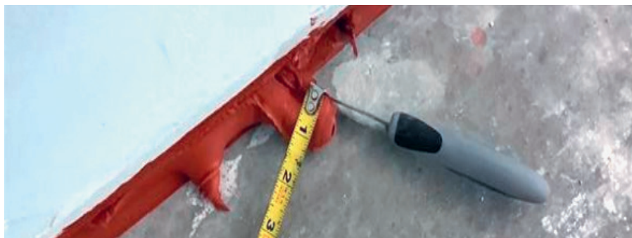
Fig. 7: Sealant thickness measurement when wet
