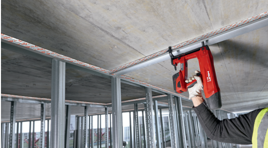
Fig. 24: Hilti CFS-TTS used on top of wall joint
