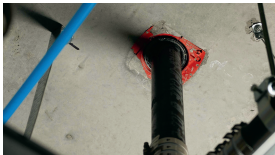
Fig. 13: Device flange should be secured to the top surface as per listed system Hilti CFS-DID
